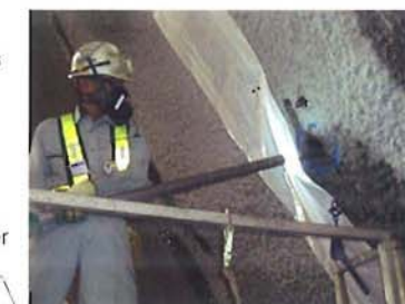
Measurements with BIP systems (The front investigation of the tunnel)
